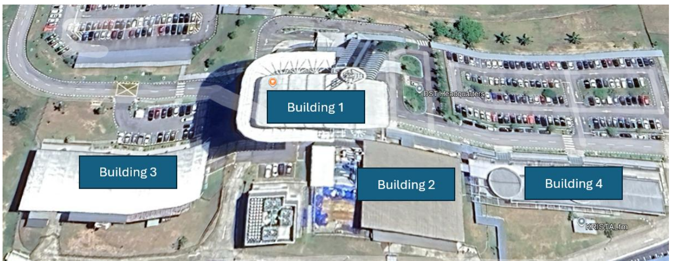
Fig 2.0 Mutiara Exchange as viewed through Google Earth.
