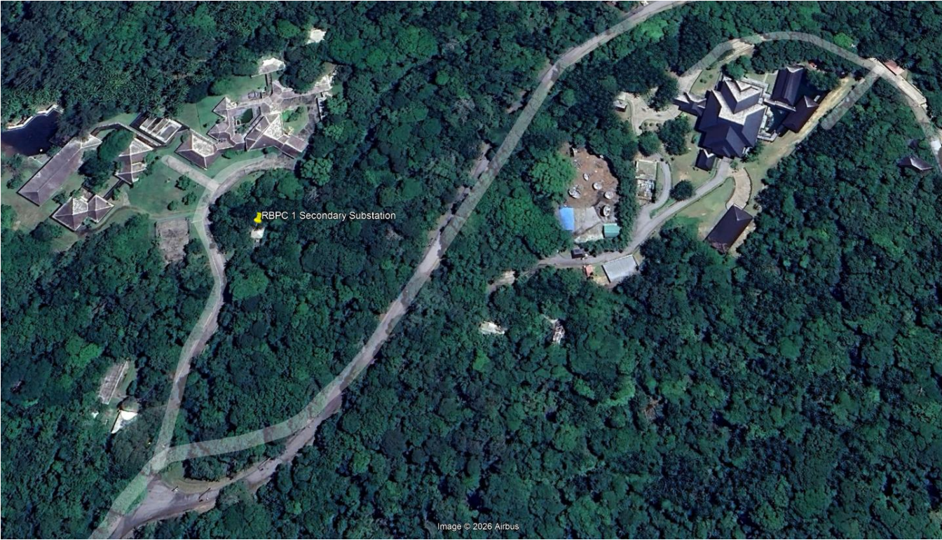
RBPC 1 Secondary Substation
