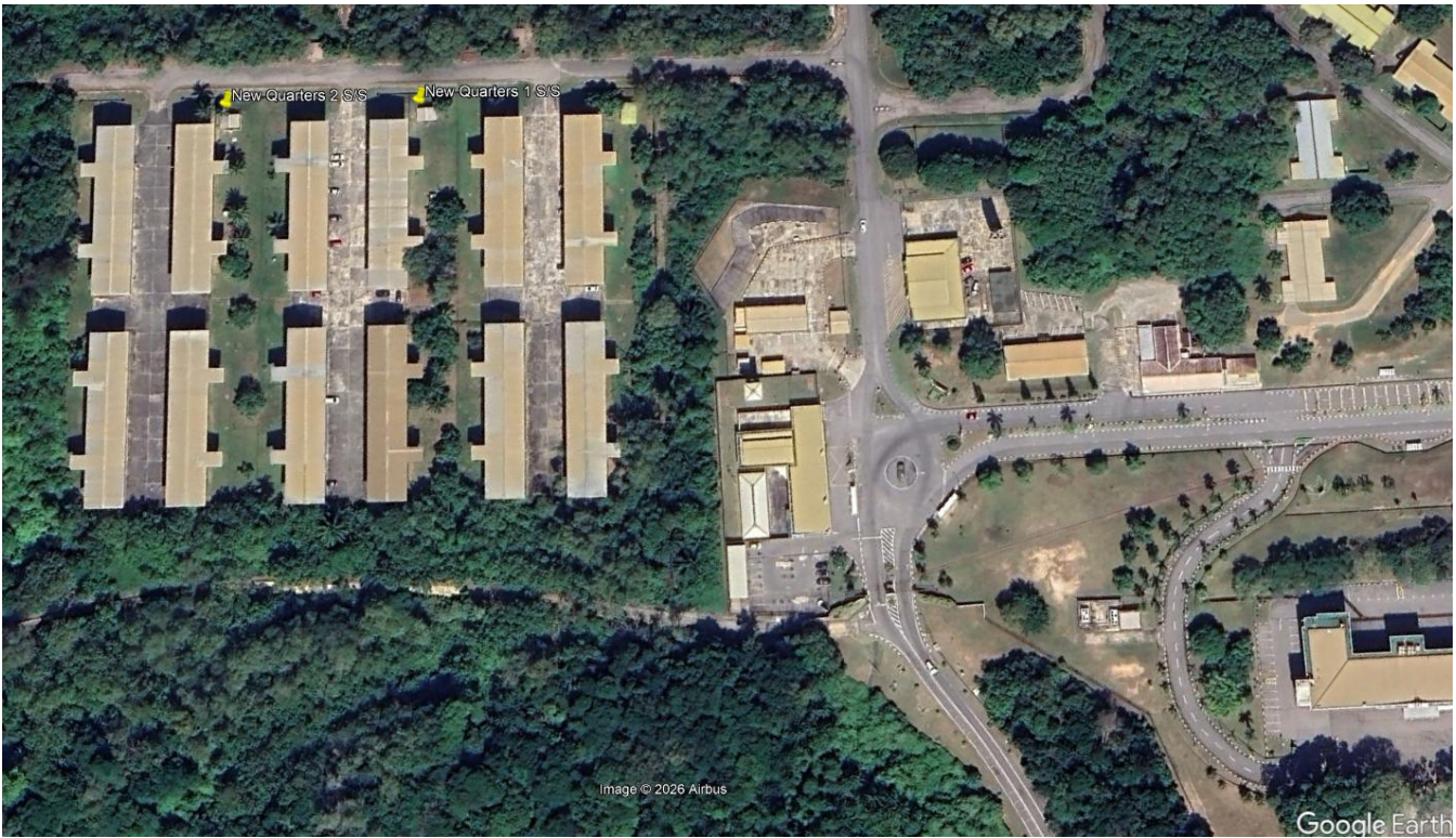
New Quarter #1 and #2 Secondary Substation
