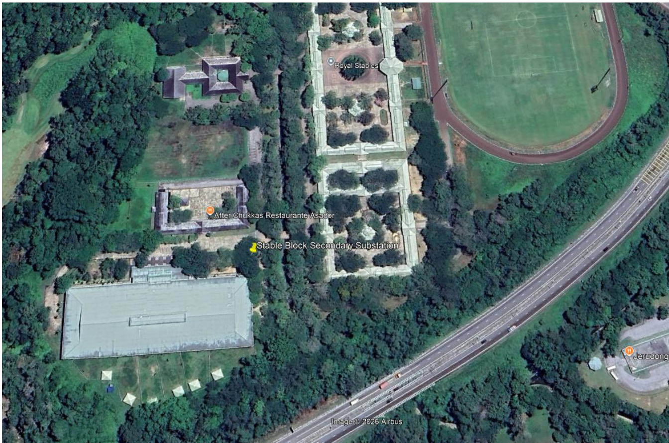
Stable Block Secondary Substation
