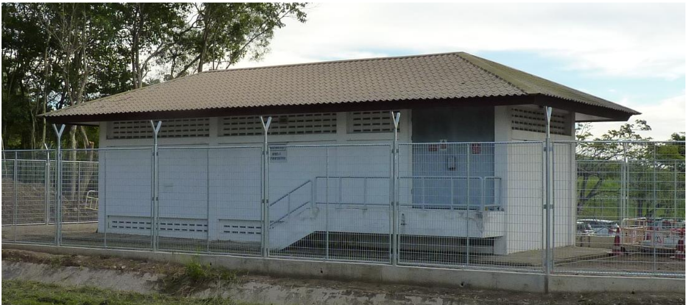
AIRPORT 5 11KV PRIMARY SUBSTATION
