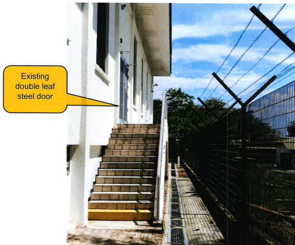
Figure 1 Existing double leaf door location
