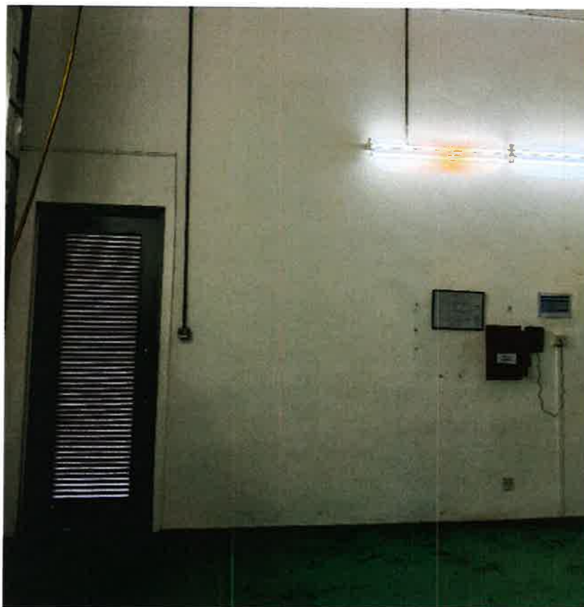
Figure 5 Internal View of Switchgear Room at the Existing Single Leaf Door Location
