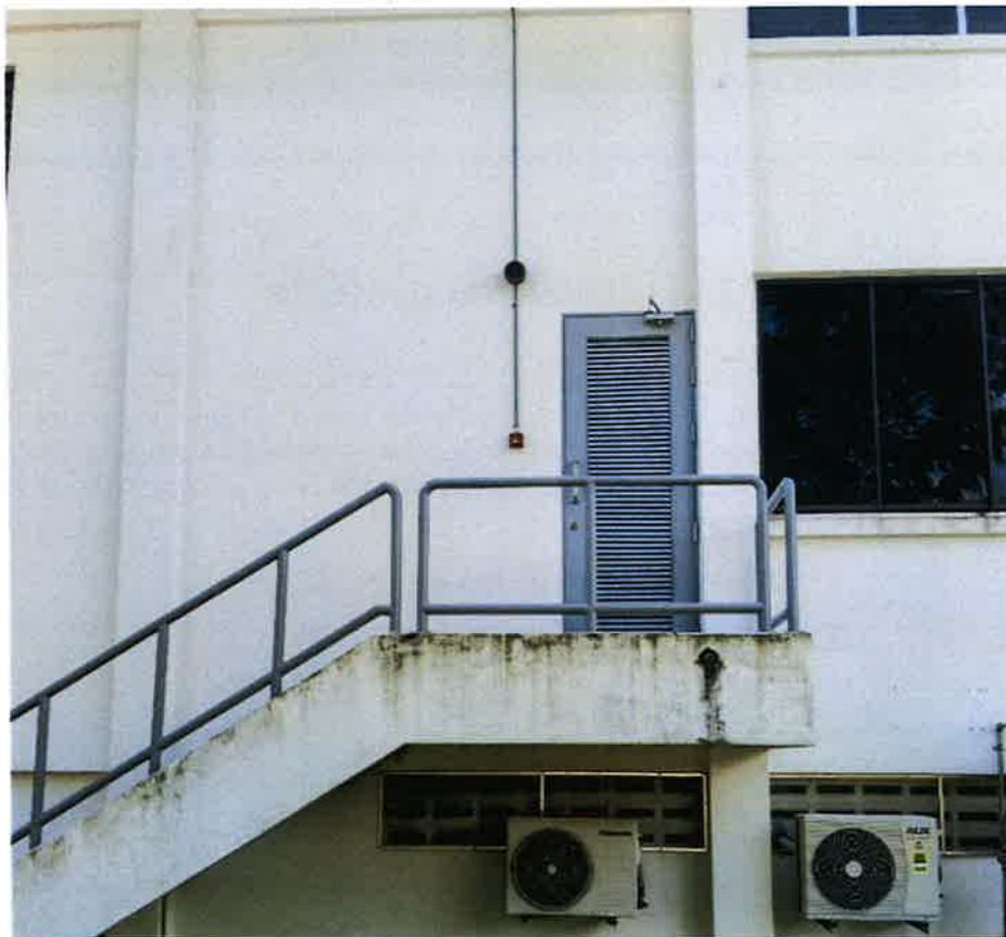
Figure 4 External View of Existing Single Leaf Door (Proposed for Conversion to Double Leaf Access Door)
