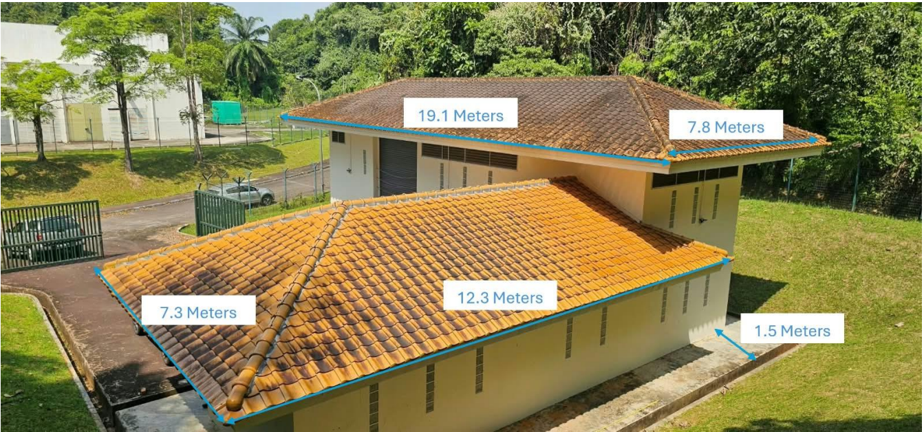
EXISTING ROOF PJT 11KV PRIMARY SUBSTATION
