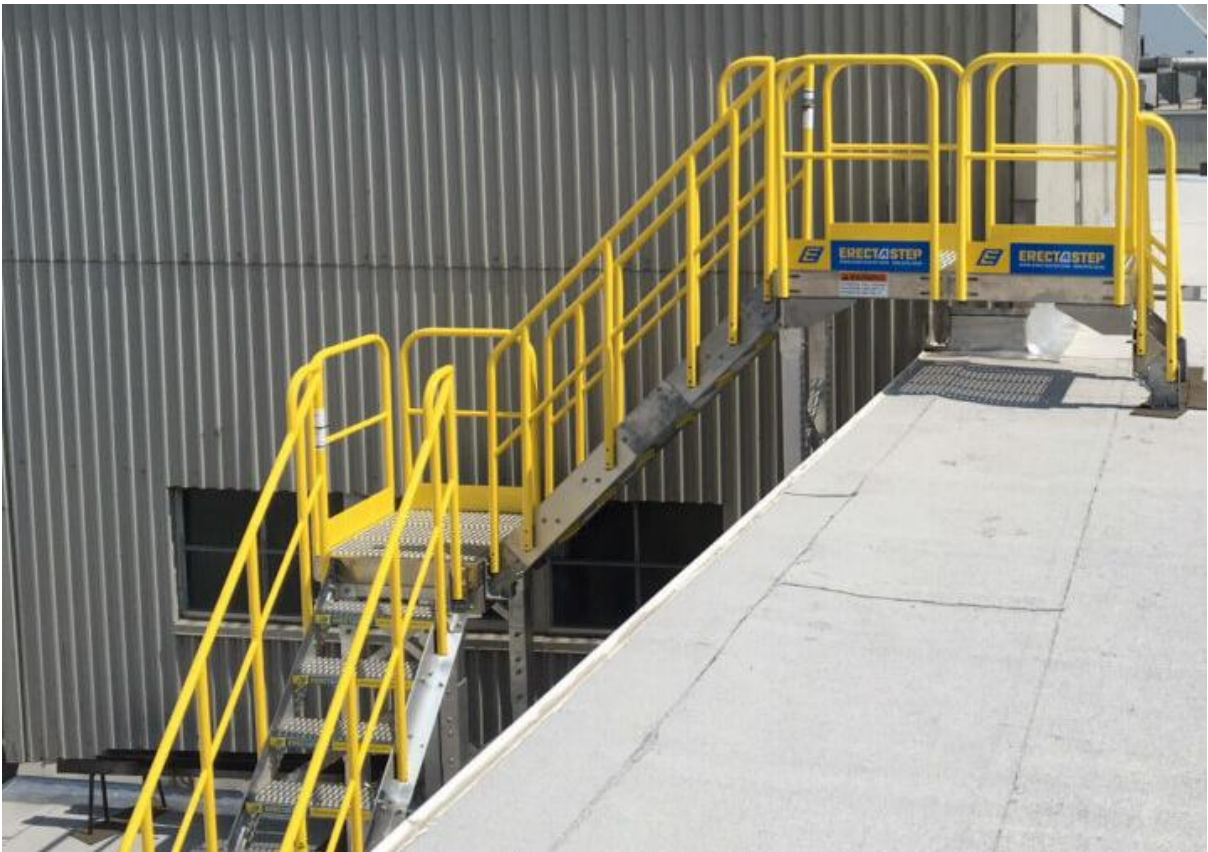
ROOF ACCESS STAIRCASE SYSTEM
